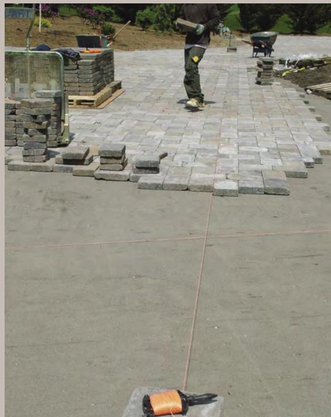
structure. Edge restraint should rest on the compacted aggregate base and contain the sand and maintain the position of the paving stone.
